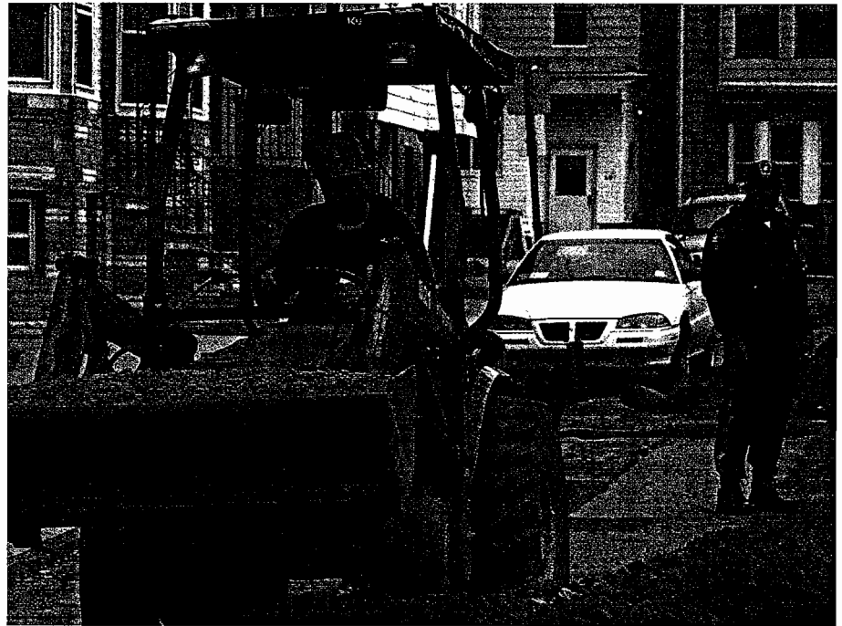
A Kearny police officer stands watch to make sure a backhoe operator from PSE&G's Harrison gas shop works safely while servicing a gas main on a busy street in Kearny, NJ.
